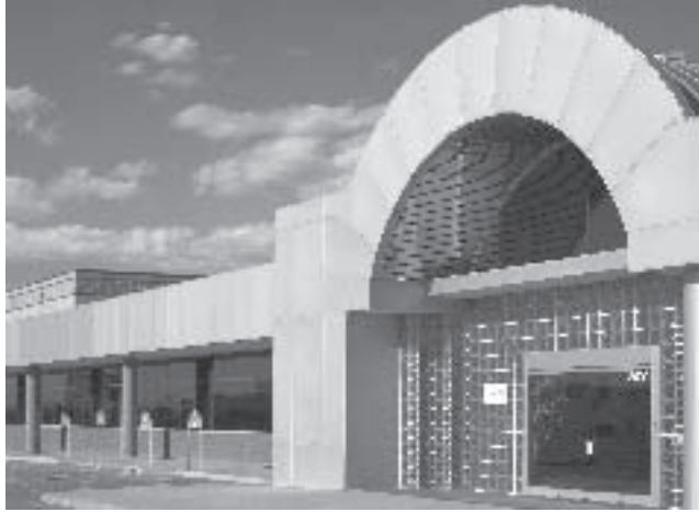
THE AMTECH SYSTEM CORPORATION (“AMTECH”) 74,000-SQUARE-FOOT OFFICE/LIGHT INDUSTRIAL MANUFACTURING FACILITY IN ALBUQUERQUE, NEW MEXICO WAS PURCHASED BY CPA ® :14 FOR $6.1 MILLION.
